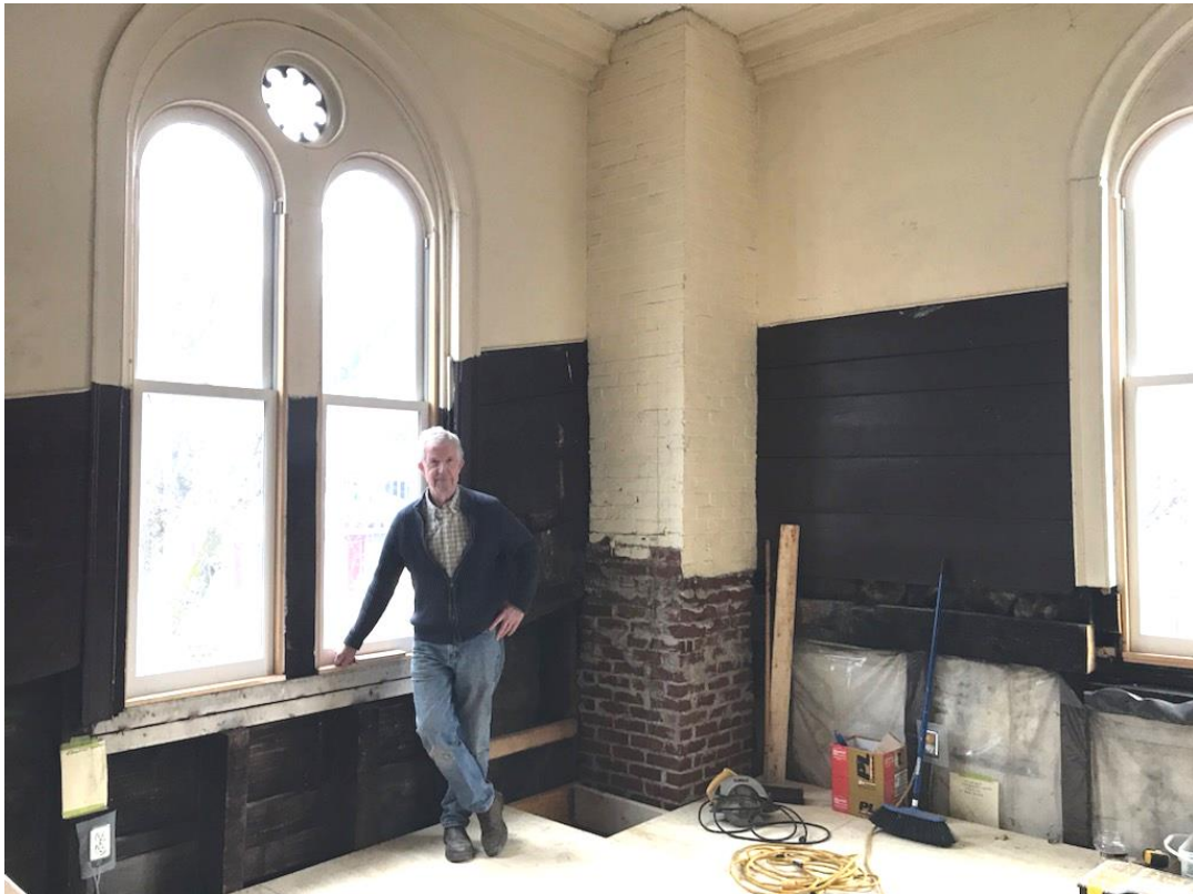
(above: Head Carpenter Ross Evans during the 2020-21 Archives Renovation Project)
